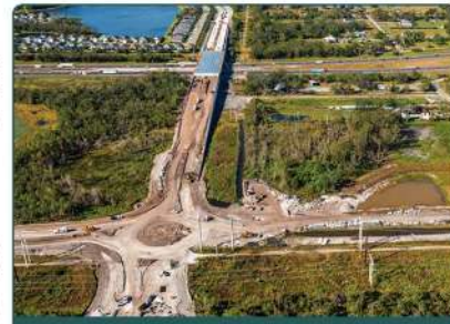
Western-facing view of construction from east of I-75
